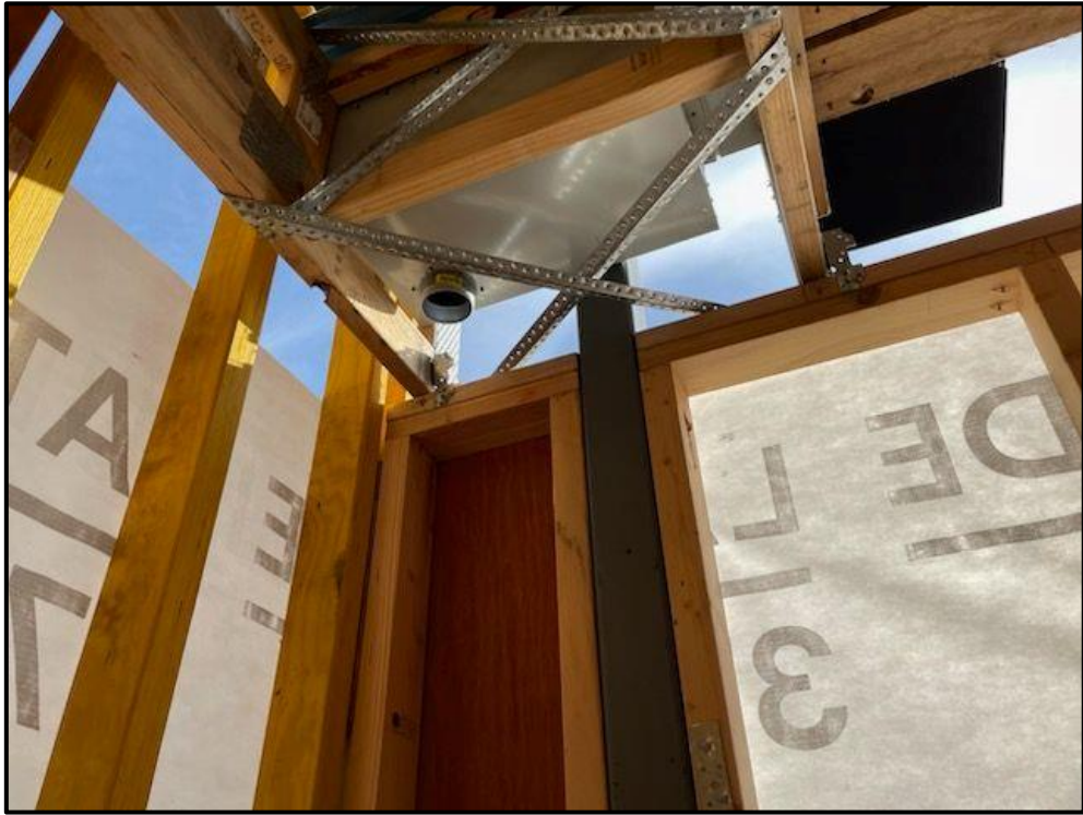
Photograph 7 – Type A overflow
