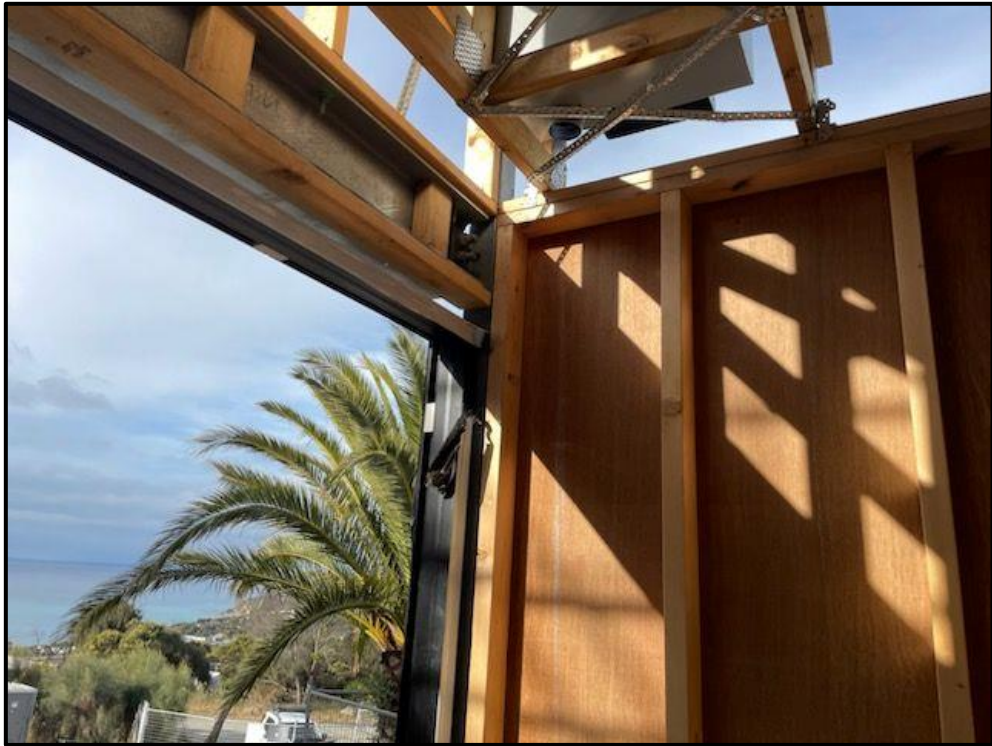
Photograph 8 – Type A overflow
