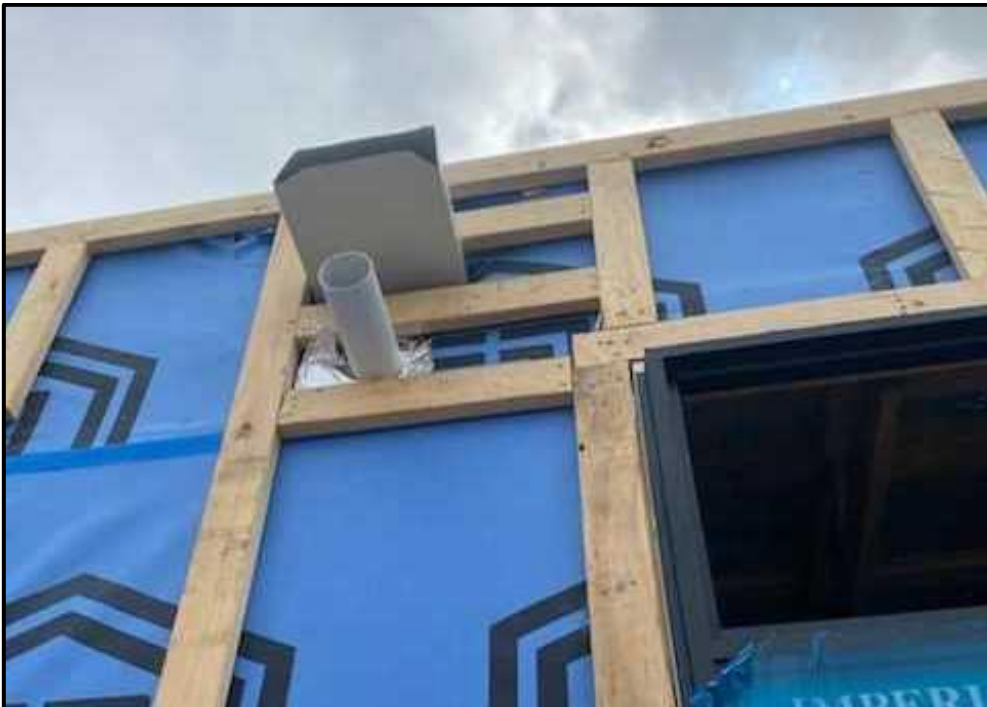
Photograph 10 - Type B overflow
