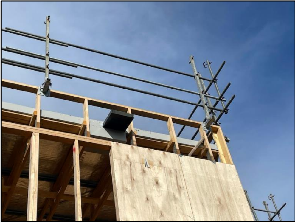
Photograph 1 – Type A overflow
