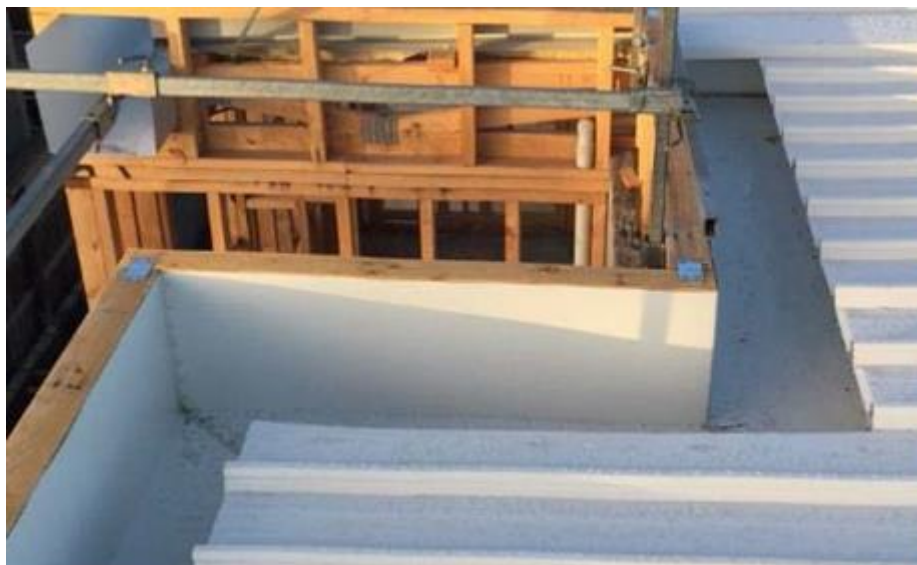
Image 2: Depicts a box gutter with a change of direction.
