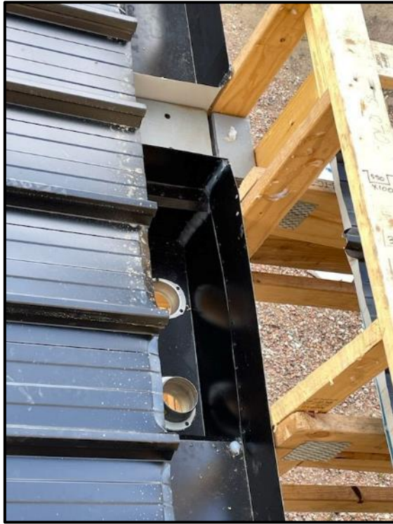
Photograph 11 – Type B overflow
