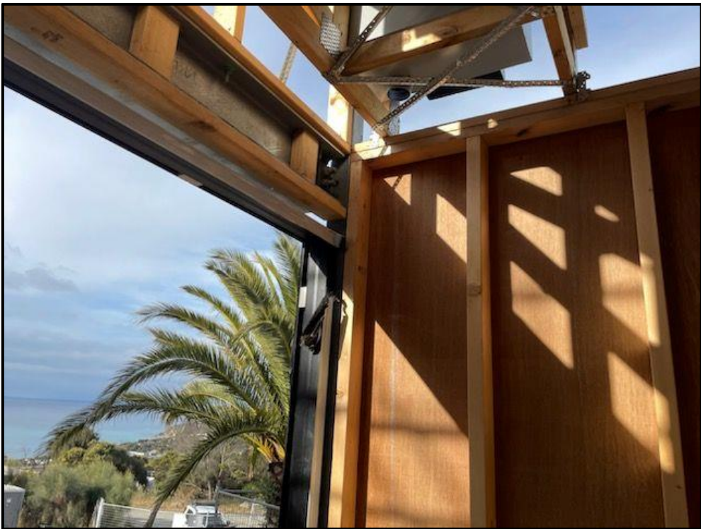
Photograph 8 – Type A overflow
