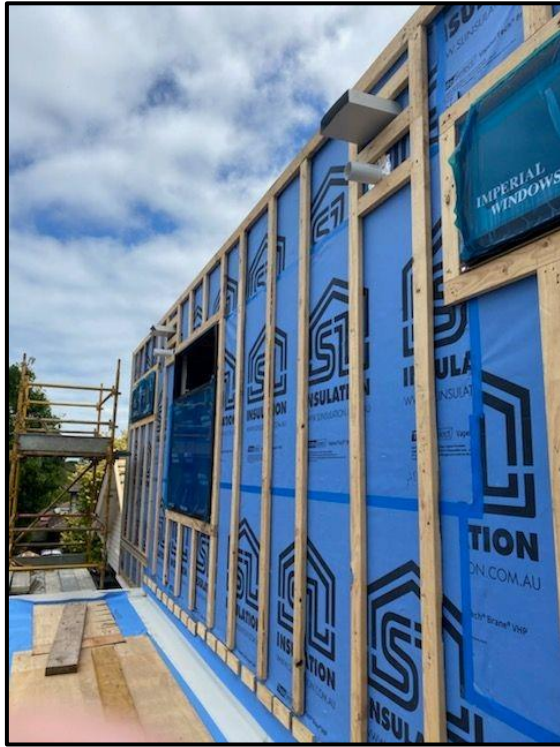
Photograph 9 – Type B overflow
