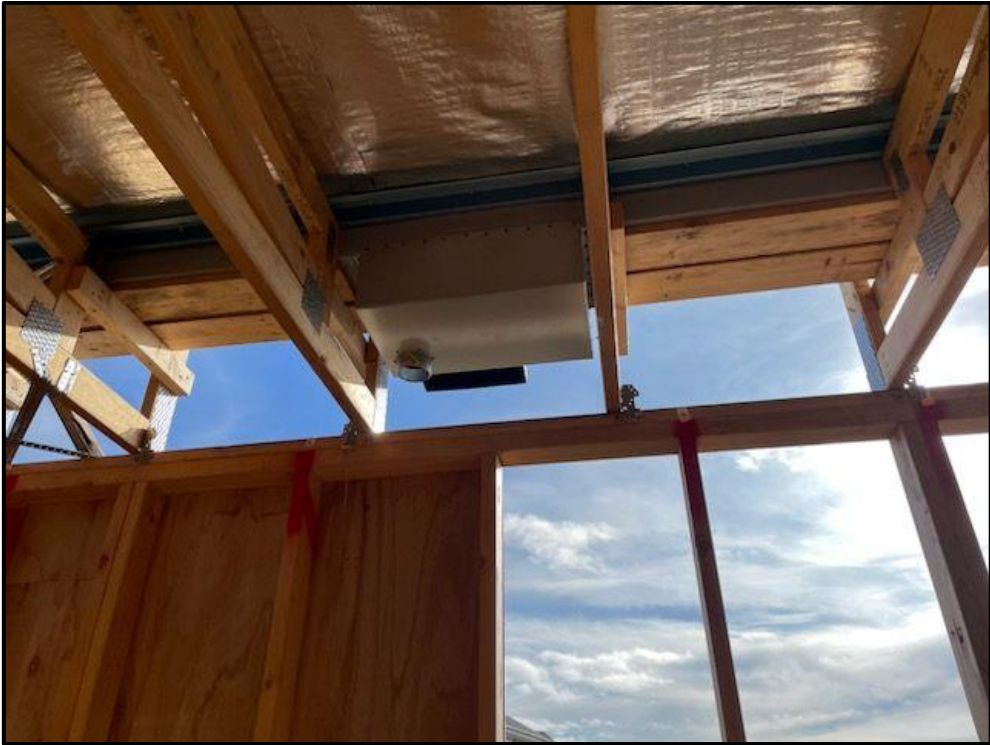
Photograph 2 – Type A overflow
