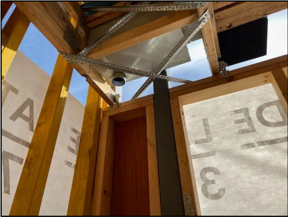
Photograph 7 – Type A overflow
