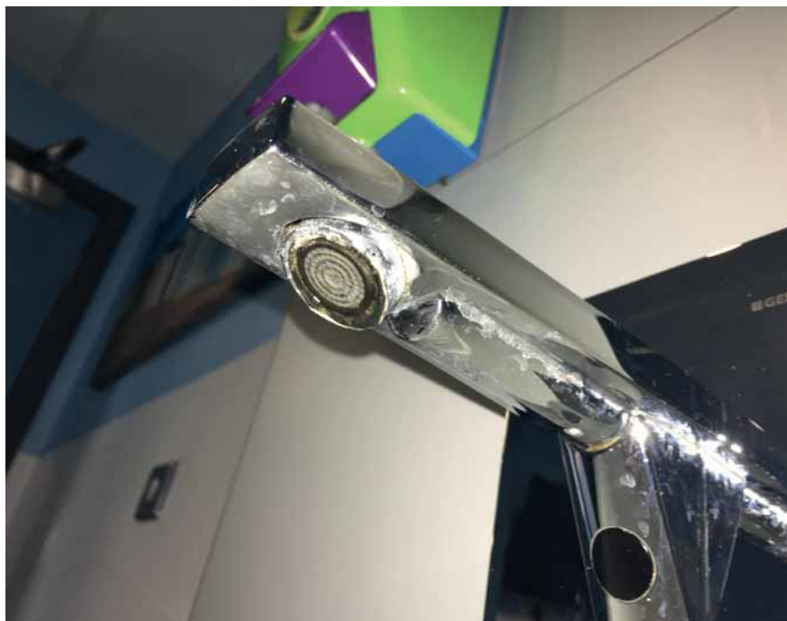
This photo clearly shows a potential pseudomonas/Legionella infected infrared basin spout and aerator.
