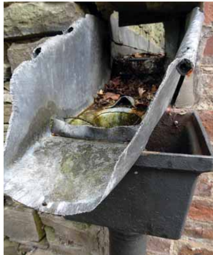
An old English rainhead design that incorporates a step down from the sole of the box gutter behind.
