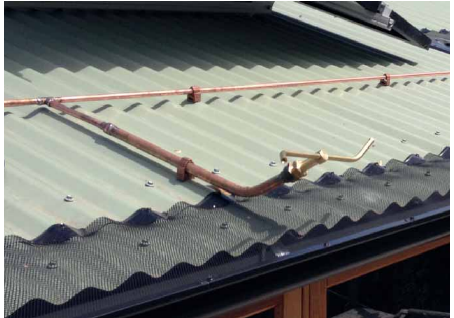
A roof mounted sprinkler system constructed of copper pipe is an ideal solution for homes in bushfire prone areas.
